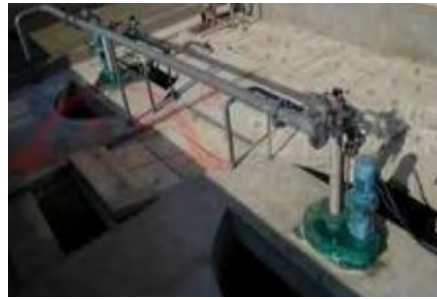
Aeration swirling grit
