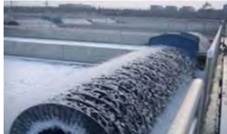
Oxidation ditch aeration turntable
