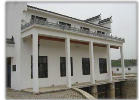
lift pump room
