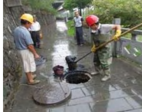
pipeline inspection well
