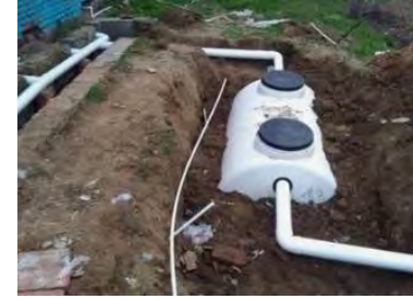
Leakage and overflow of household treatment tank
